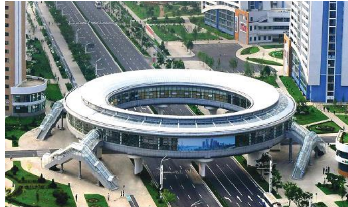
The viaduct in Songhwa Street
