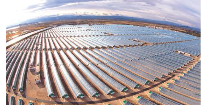
Modern, large-scale Ryongpho Greenhouse Farm built in 2022 in the northeastern part of the country
