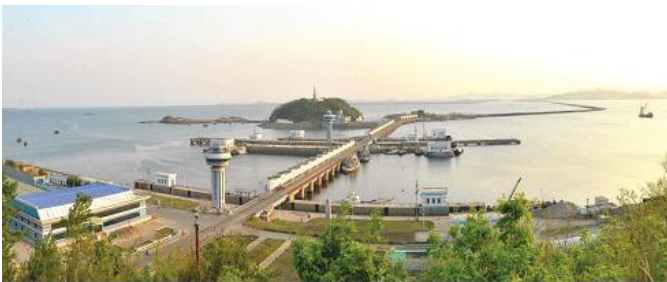
West Sea Barrage built in 1986 across eight kilometres of wild sea in the short period of five years
