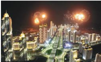
Part of the first-stage 10 000 flats in Songgho 1st set built only in a year pursuant to the construction plan of 20 000 flats in Pyongyang (2012)
